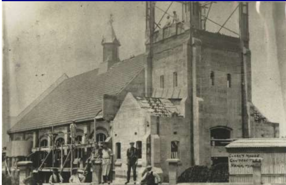
Above: Construction of the church
